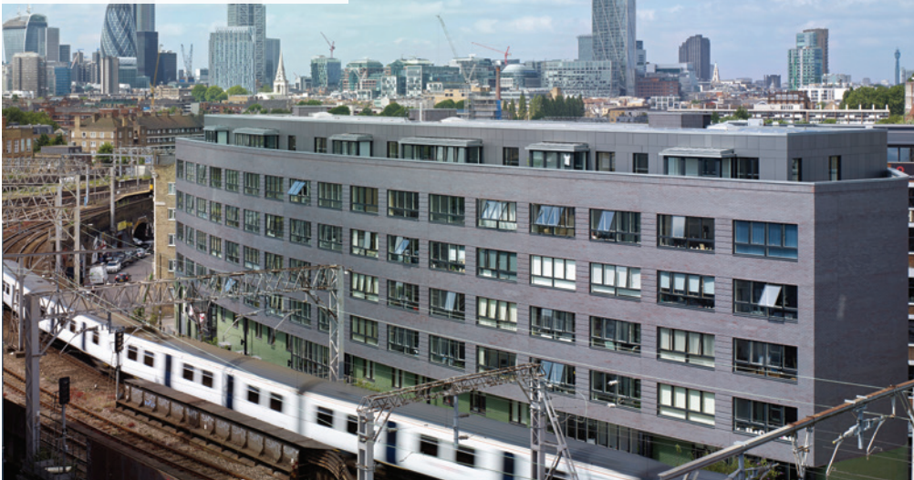
Mint Street, Bethnal Green, is a new housing block and public street for Peabody in London's East End, adjacent to a noisy railway
